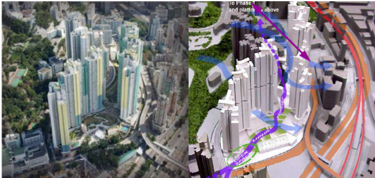
Fig. 2 (left) A bird's eye view of the Upper Ngau Tau Kok Estate redevelopment project. (right) physical model with the design concept of introducing wind while fencing out traffic noise. Source: Hong Kong Housing Authority [17]s
